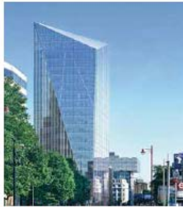
4) 240 Blackfriars Road Architect: AHMM Roof Height (AOD): 89m Roof Height (AGL): 80m Total Floors (O.G): 18 Program: Mixed-use
