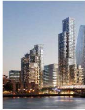
5) Sampson House & Ludgate House Architect: PLP Architecture Roof Height (AOD): 169.6m Roof Height (AGL): 165.6m Total Floors (O.G): 48 Program: Mixed-use
